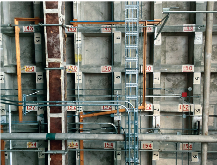
The ceiling at the No. 1 Supply Depot, showing tracks for the internal train that moved materials around the building and coordinates to locate them
