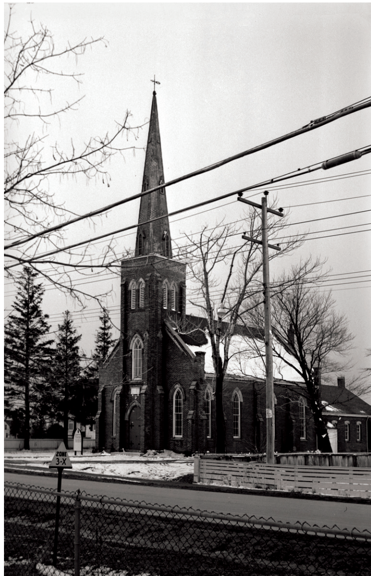
Downsview Church on Keele Street, 1954
